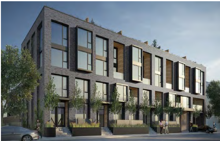
South Façade Credit: Zinc Development
